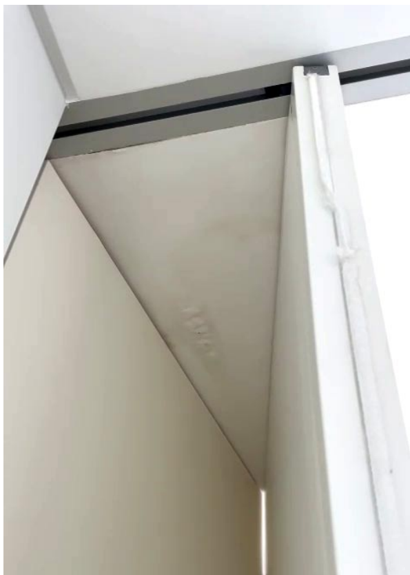
Bulged sliding doors in the kitchen.
