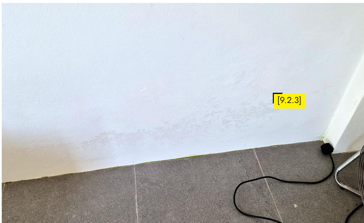
9.2.3. Crumbling plaster, soggy paint coming off.
