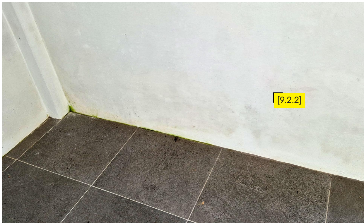
9.2.3. Crumbling plaster, soggy paint coming off.
