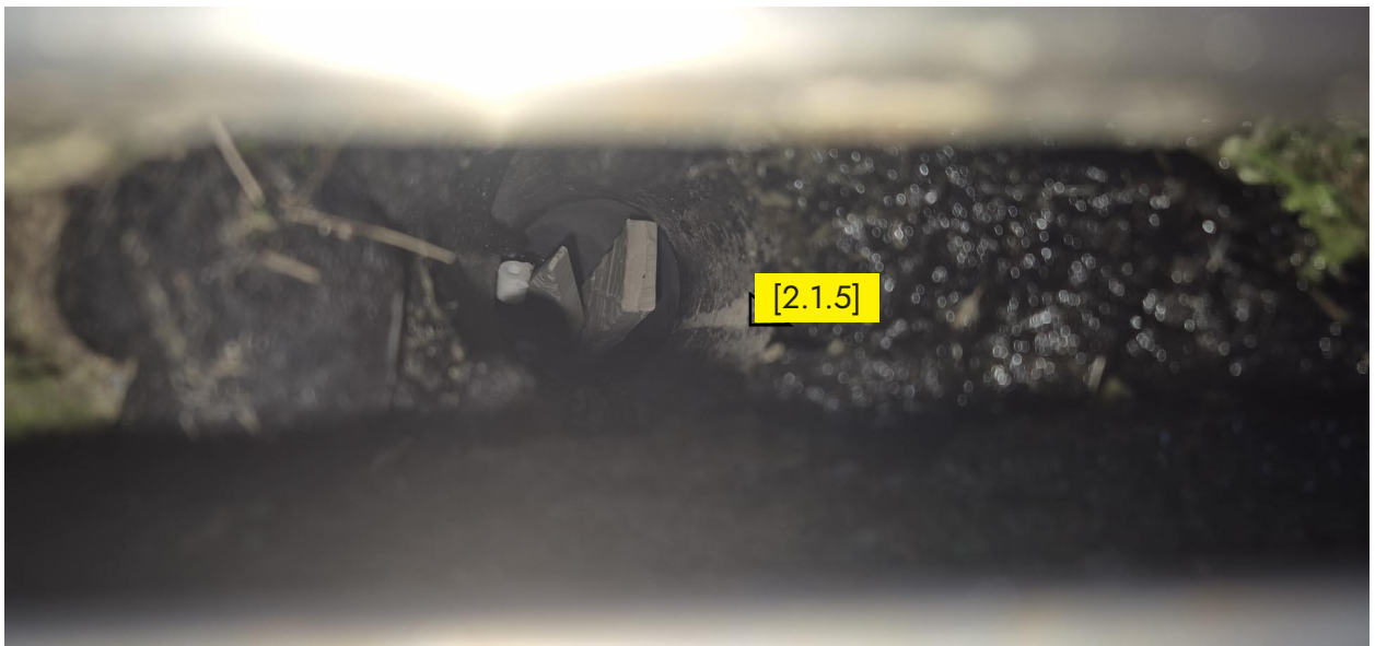
Endoscopic image of the debris in the terrace drainage pipe
